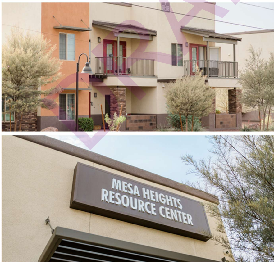
Figure A-1. Mesa Heights Apartments & Resource Center
