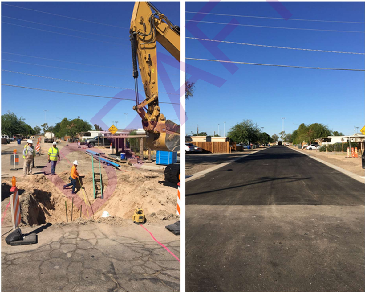
Figure A-3. Harvard Street Sewer & Road Project
